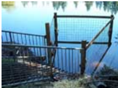
The complete installation.
