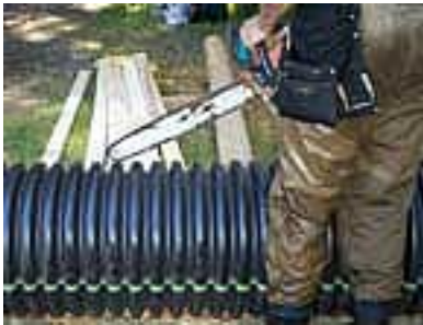
Cutting holes in the pipe
